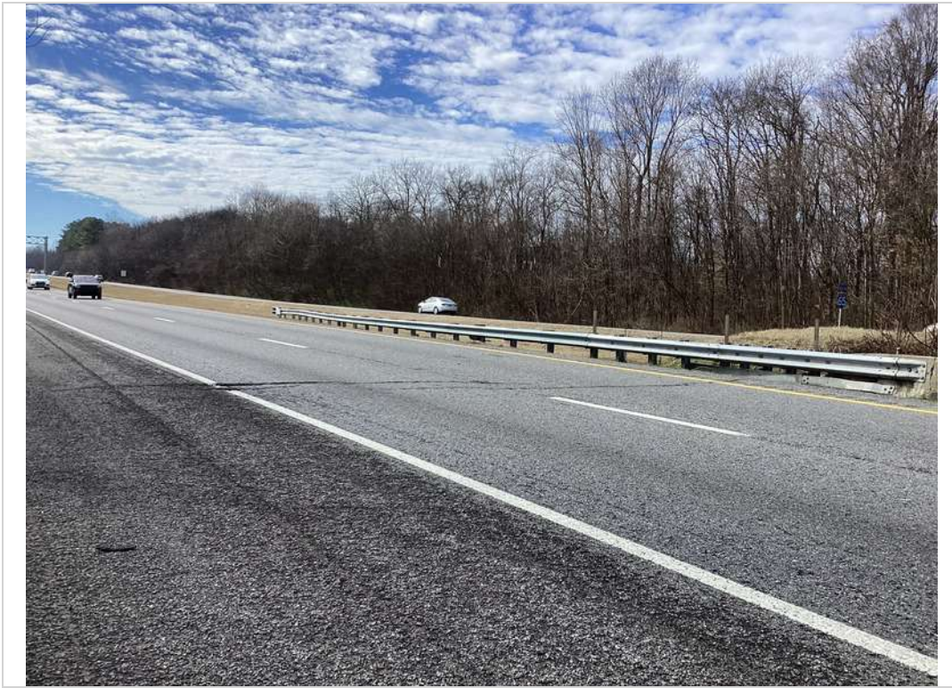
Approach 1 looking back
