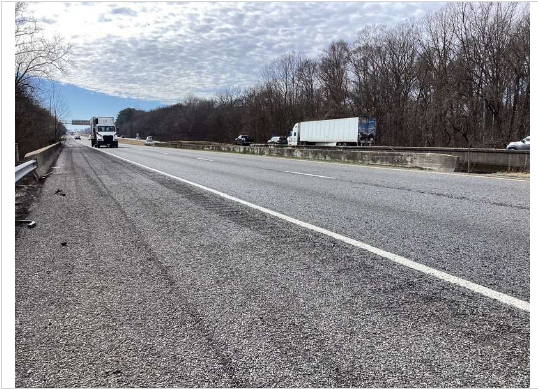
Approach 2 looking back
