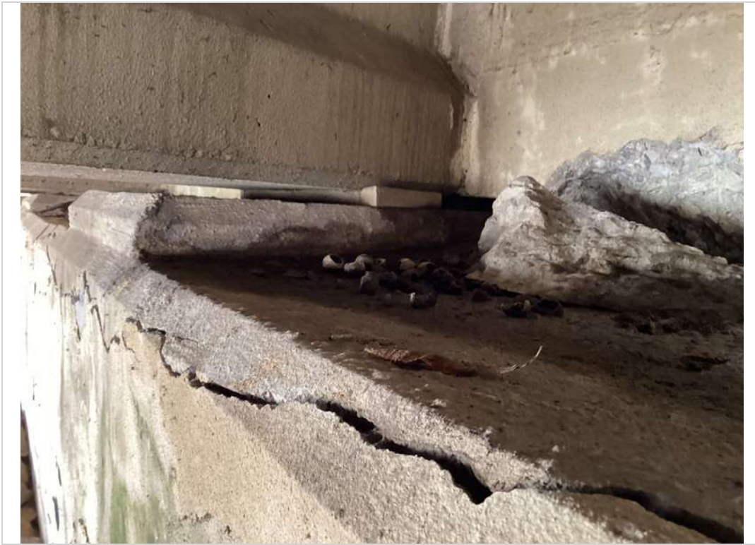
Typical abutment bearing pad
