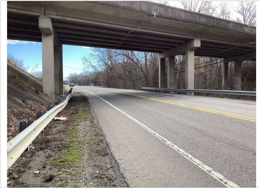
Looking back on underpass route
