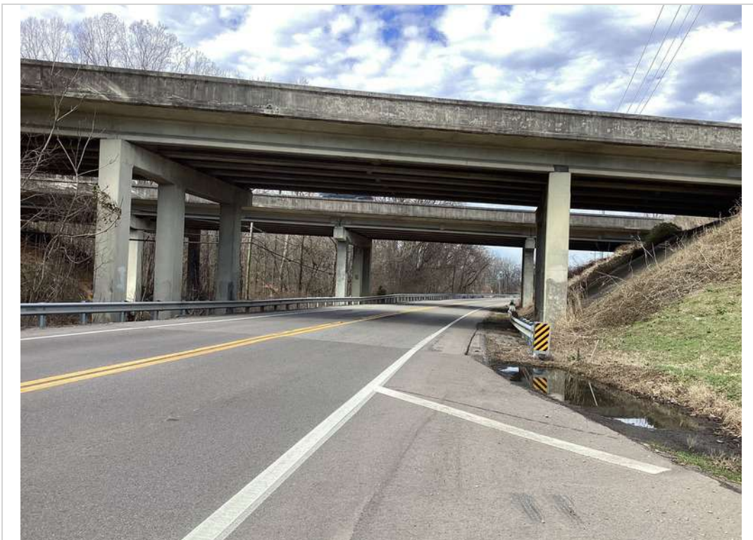
Looking ahead on underpass route
