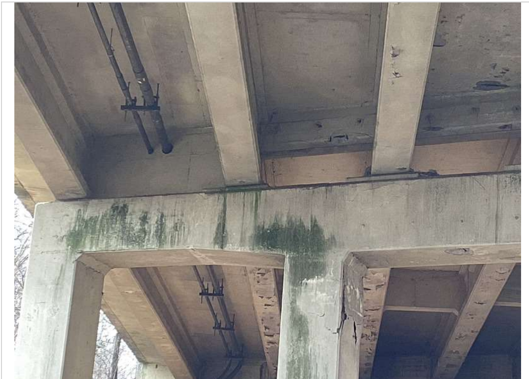
Moderate cracks in caps of bent typical
