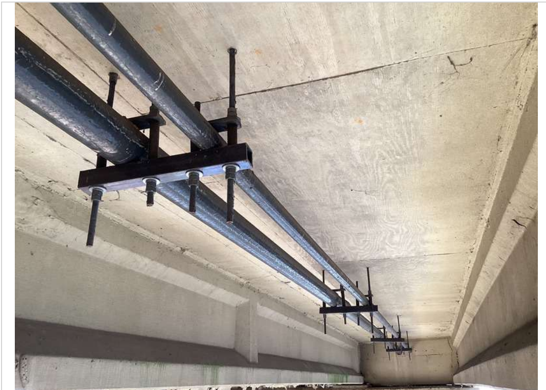
Utility line in Bay E typical all spans
