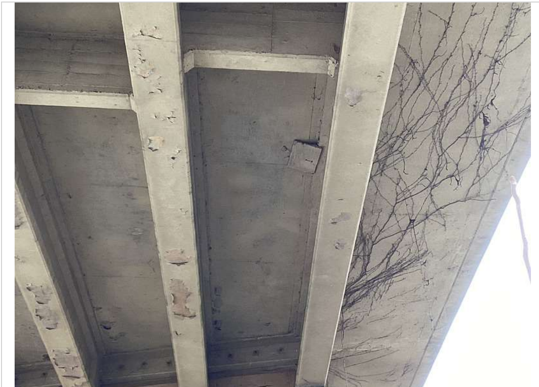
Span 2 Bay A patch with formwork still present. Typical patch for Span 2
