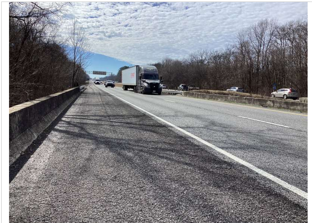
Top of deck looking back
